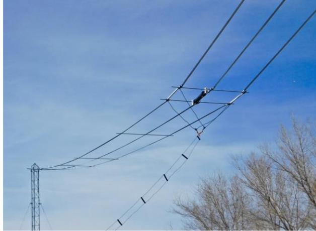
Moving to Carson Valley was an antenna challenge, so he constructed a 120-foot antenna called a "T3FD" (terminated three-wire folded dipole) using one inch wide Electric Fence Poly Tape. The tape has seven aluminum wires running through it, although stainless steel wire is available.
