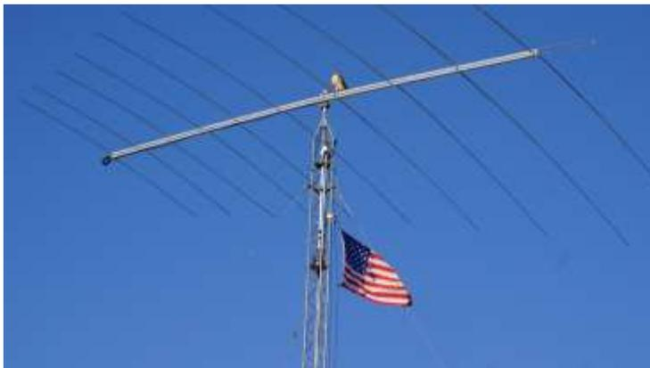
When Jim Marshall K6LR got home from Eagle Lake, he noticed his log periodic antenna was pointing west. The rotator controller said it was pointing east. He also found that turning the rotator did not move the antenna. He determined the rotator coupler had given up after four years. (*Ed Note: With the winds we have around here, it's amazing the antenna stood up this long.*)
